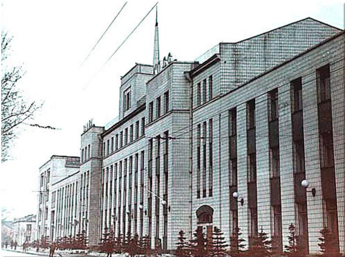
The LOMO PLC Works at Chugunnaya Street in St Petersburg. Picture from 1962
