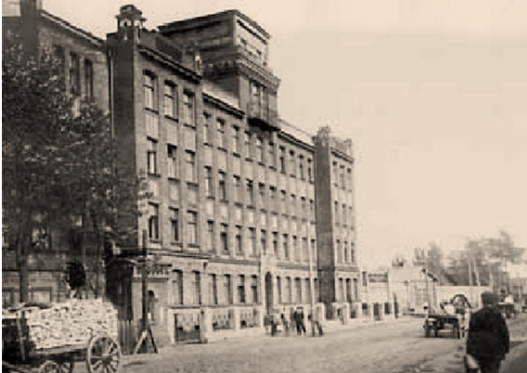
The LOMO PLC Works at Chugunnaya Street in St Petersburg. Picture from 1914
